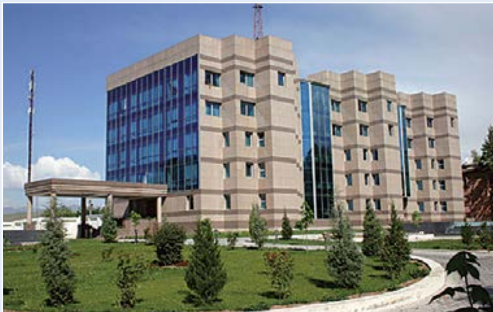
The National Bank of Tajikistan Administration building
