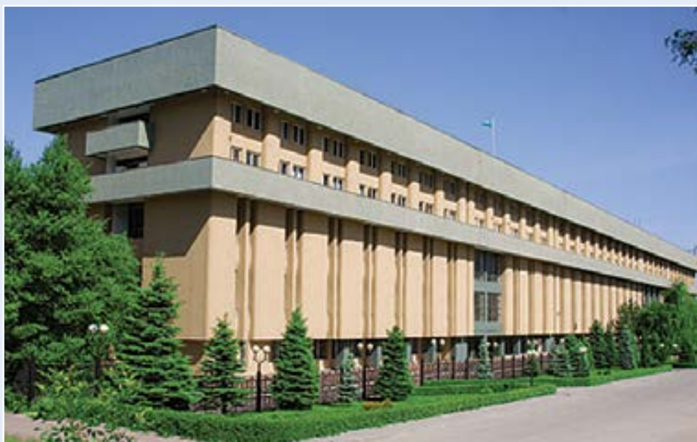
The National Bank of the Republic of Kazakhstan Administration building
